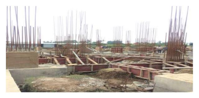
In Block A2: Pile Cap Plinth beam Shuttering work in progress.
