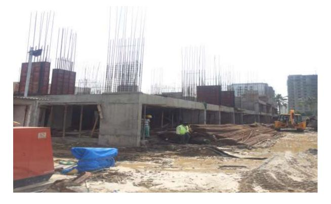
In Community Hall: Excavation, Pile cap Concrete casting, pile chipping &Column Casing work on progress.
