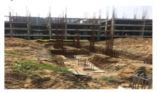
In Block D2 : Fourth floor level slab 2nd half Shuttering & Bar Bending work on progress.
