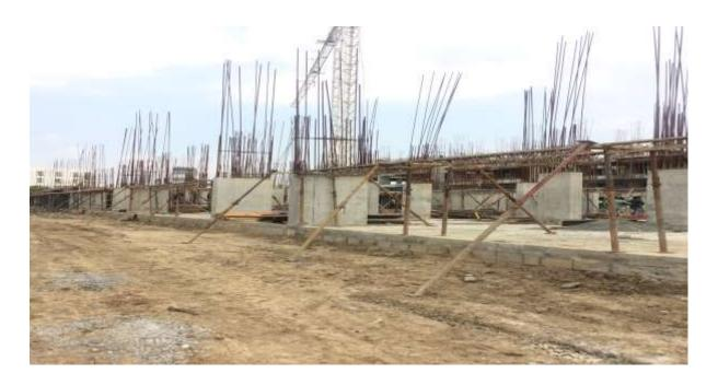
In Block D1: Excavation, Bar bending & Shuttering for Pile cap work on Progress.
