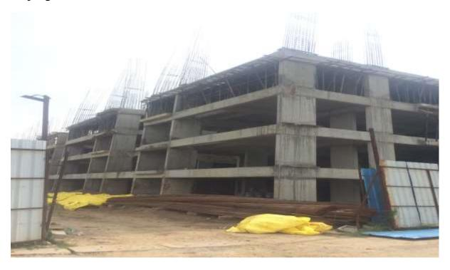
In Block D3: First floor Column Shuttering and Bar bending Works in Progress.
